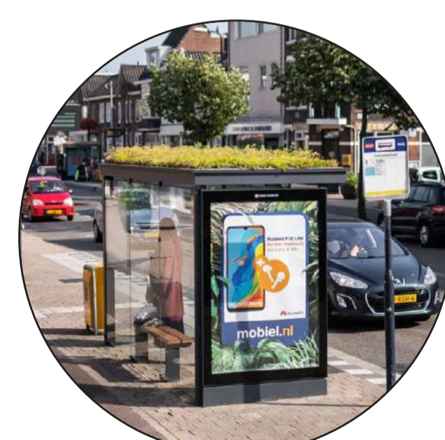
Green roof bus stop
