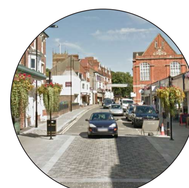
Raised table crossing to improve connection of site
