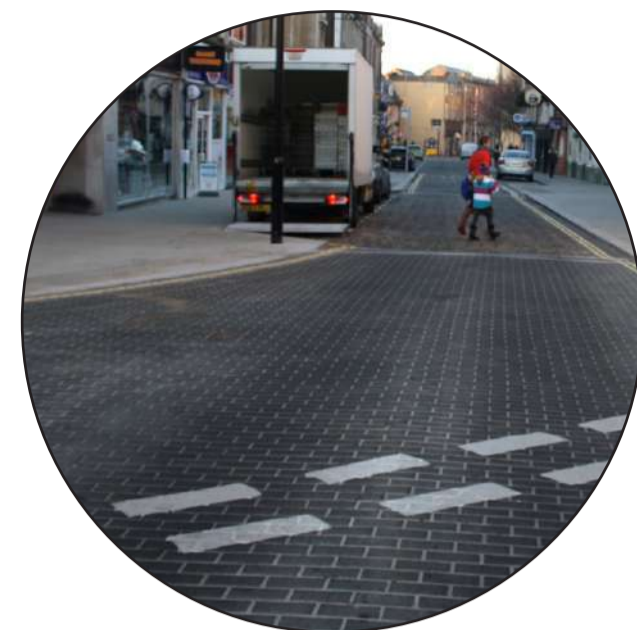
Raised table at junction
