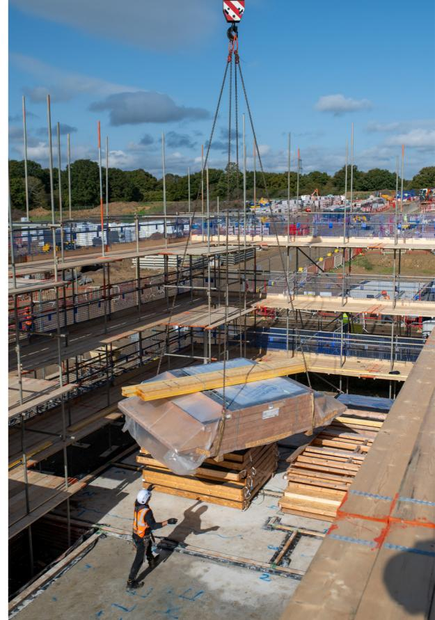
An image of the timber frames being installed at the Vistry site. A crane can be seen lifting the timber into place
