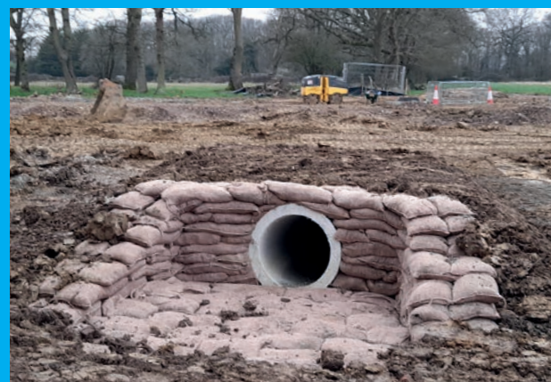
Left: A drone shot looking northeast shows the roundabout with the A2300 and part of the site of the future Centre for Outdoor Sport Right: a mammal crossing is installed to enable animals to cross safely once the road is built
