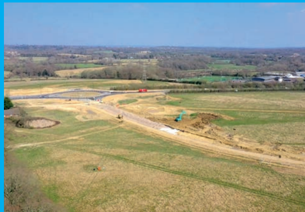
Left: A drone shot looking northeast shows the roundabout with the A2300 and part of the site of the future Centre for Outdoor Sport Right: a mammal crossing is installed to enable animals to cross safely once the road is built
