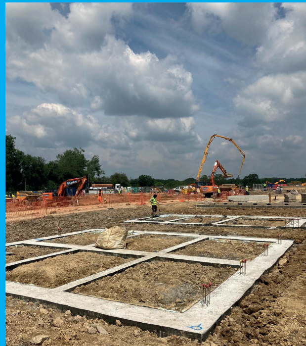
Foundations for houses at Freeks Farm
