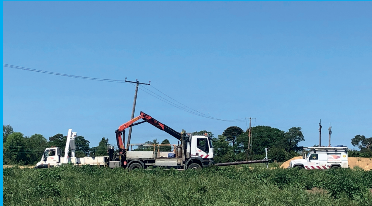
UK Power Networks conducting overhead line works at the Sisk site
