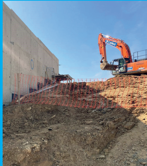
Work on the bridge over the River Adur
