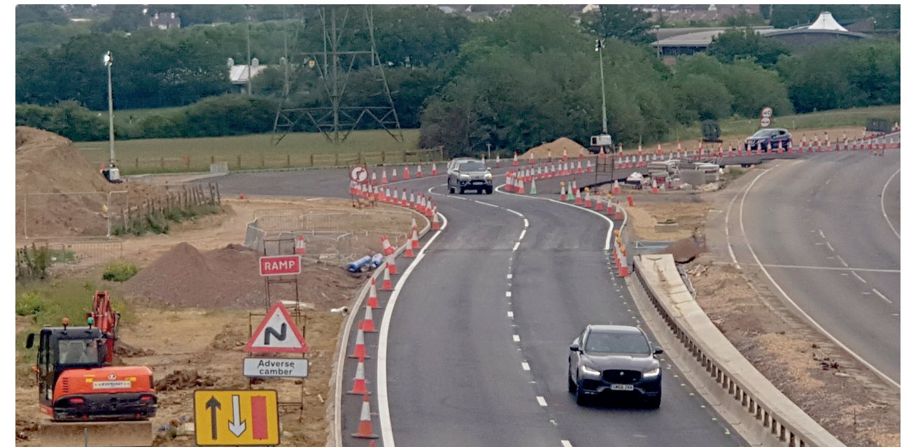
The Western Link Road under construction
