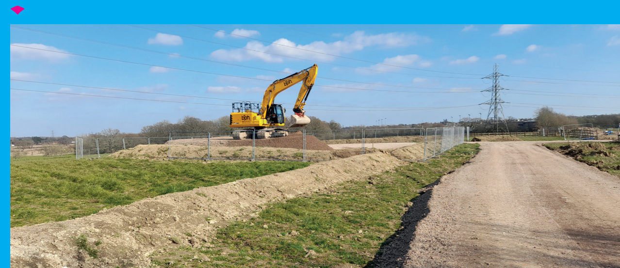
Jackson Civil Engineering begin work on the Western Link Road
