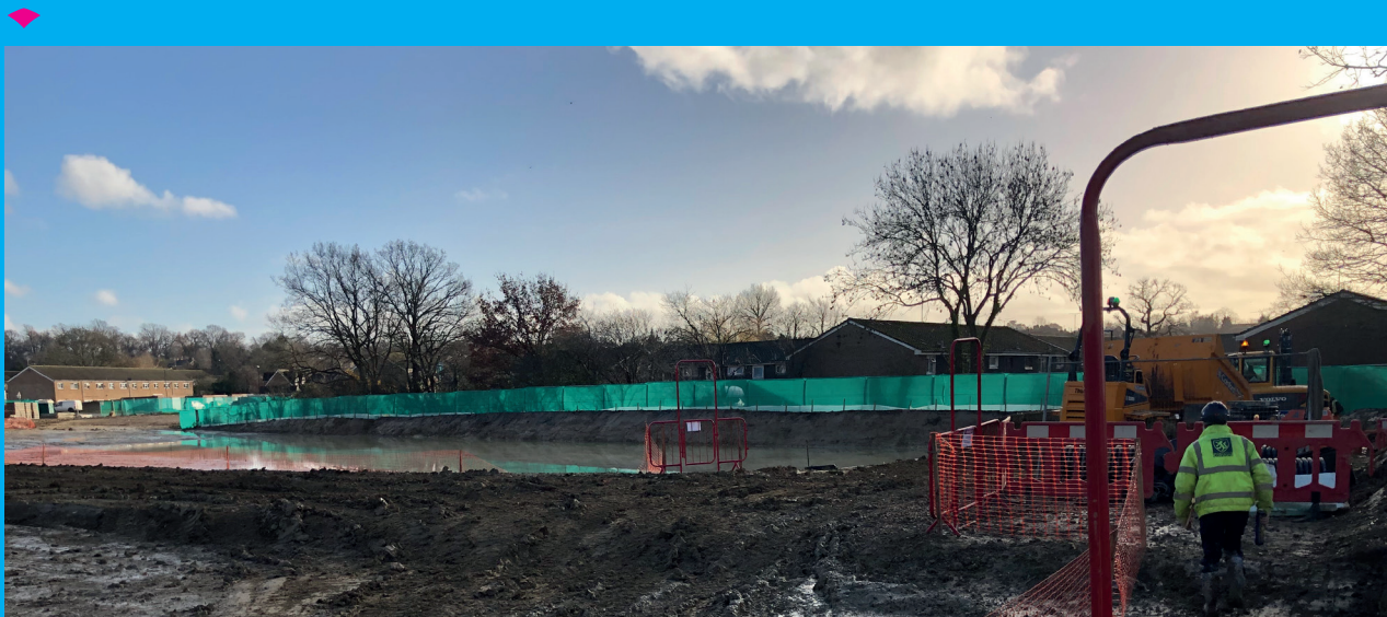
View of the new access road under construction
