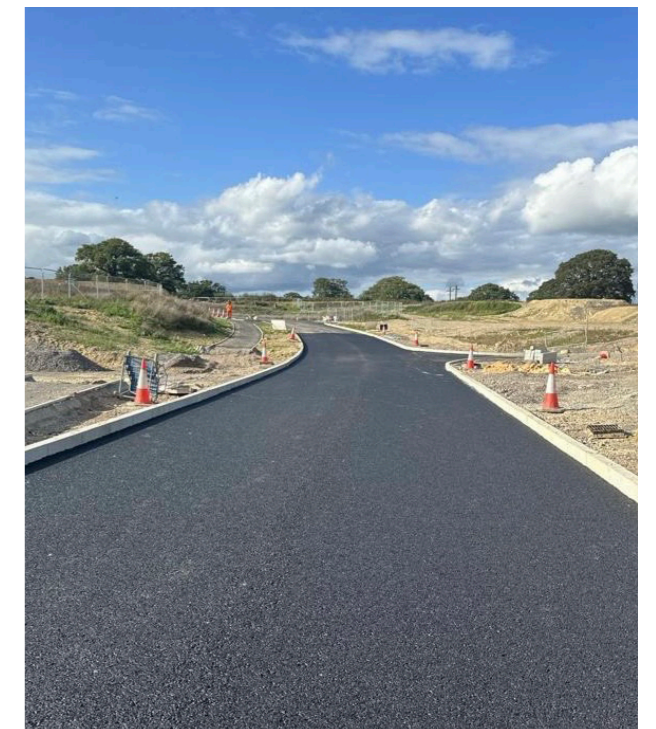
Image of the tarmacked link road
