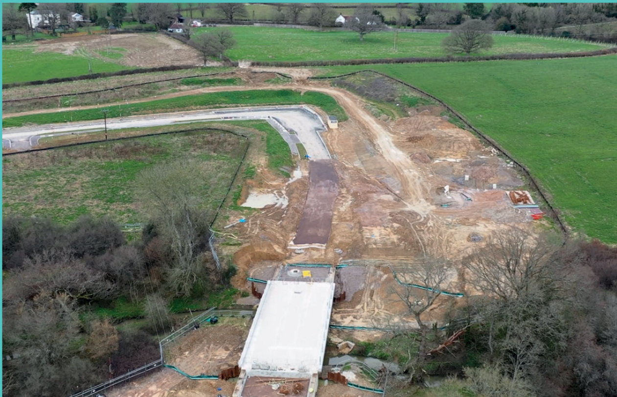
A drone image of the Eastern Bridge and Link Road
